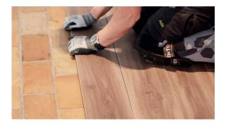
To fit the last row of panels you will usually need to cut them in. Do this as follows: lay a panel on top of the previous row with the groove towards the wall, lay another panel upside down up to the edge of the wall and mark the panel underneath. Cut the panel to size and fit the last row.
